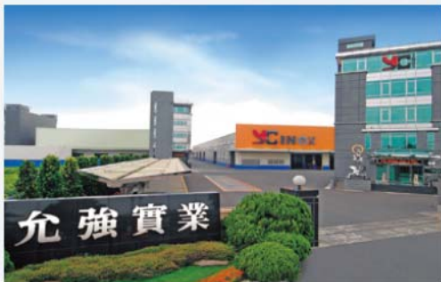
▲ TAIWAN HQ & TUBE MILL 54,000 m 2
